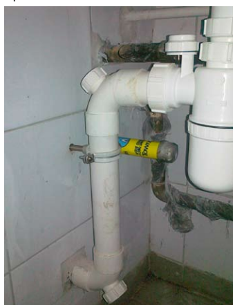
Picture 3: After the gas meter is removed, mark clearly in English and Chinese that the pipe contains gas
