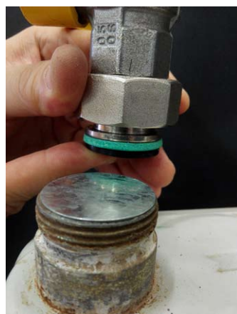
Picture 1: Add a piece of meter cap-off disc to the gas inlet of the gas meter (picture courtesy of the Vocational Training Council)
