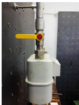
Picture 2: Turn the lever anti-clockwise to lock and fit it with a new red safety plastic cap (picture courtesy of the Vocational Training Council)
