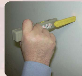
▲ 使用金屬探測器確定牆內喉管位置 Use metal detector to detect the exact position of concealed pipes and conduits.
