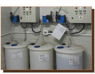
Check conditions of water treatment facilities Drain off the dead lea 檢查水處理投藥設備的狀況
