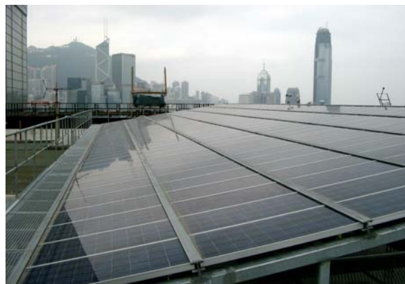
Figure 2-2: Rack Type PV System
