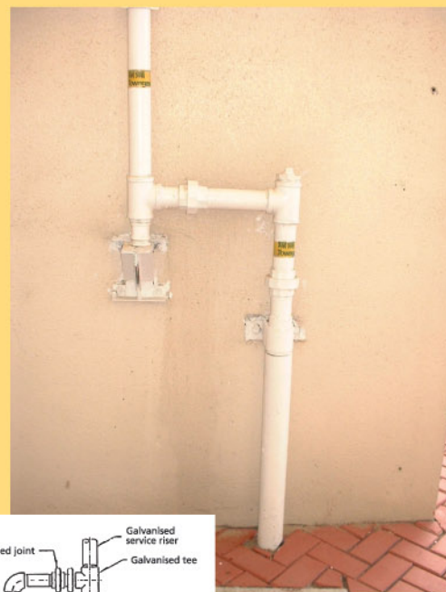
The installation of glass-fibre reinforced polyethylene risers
