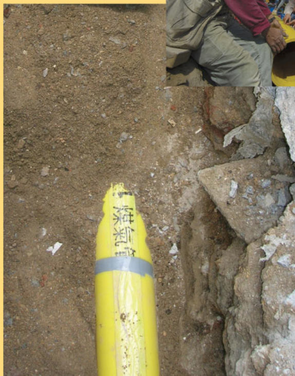
The laying of polyethylene gas pipes
