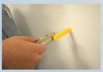
Use a metal detector to detect the exact locations of the pipes inside the wall before carrying out the work.
