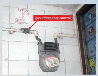
Turn off the gas emergency control to stop gas supply immediately in an emergency.
