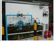
A water spray system (see photos) is also installed at the station. When LPG concentration reaches 40% of the Lower Flammable Limit, the system will be activated to prevent fire occurrence.
