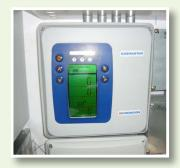
Gas detectors (see photos) are provided at different locations in an LPG filling station. In the event of LPG leakage, the system will activate an audio alarm when LPG concentration reaches 20% of the Lower Flammable Limit. When LPG concentration reaches 40% of the Lower Flammable Limit, the system will automatically give a signal to the Fire Services Communication Centre for attendance by firemen.
