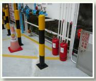
In addition to these major fire services facilities, portable dry powder fire extinguishers are provided in the filling station. Warning signs of "LPG Filling Station", "No Smoking", "No Naked Lights", etc are posted conspicuously to raise the alert of staff and customers.
