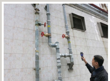
Figure 3: Checking a service pipe
