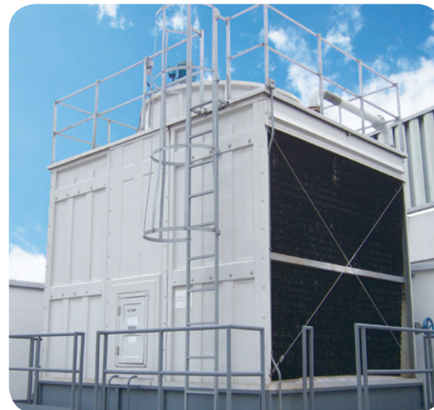
Cooling Tower Source: Electrical and Mechanical Services Department
