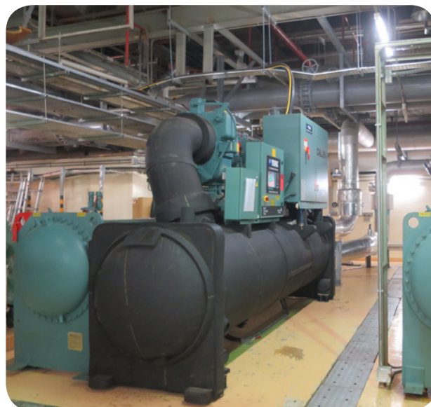
Water Cooled Chiller Source: Electrical and Mechanical Services Department
