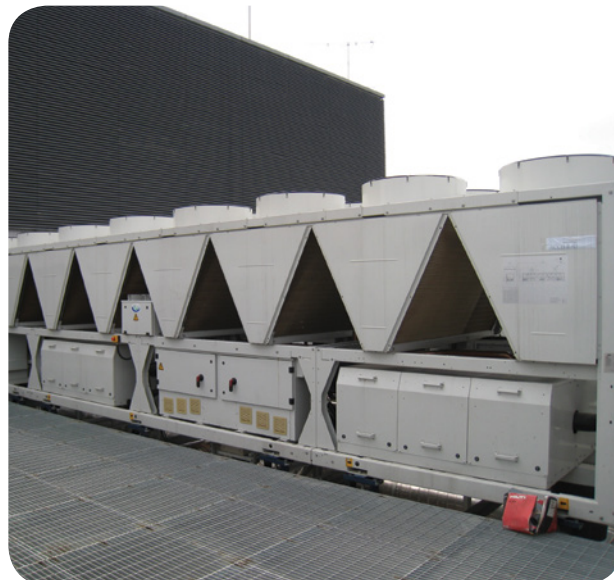
Air Cooled Chiller Source: Electrical and Mechanical Services Department
