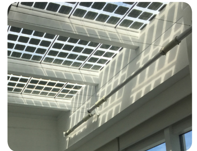
Building-integrated PV (BIPV) System Source: Electrical and Mechanical Services Department
