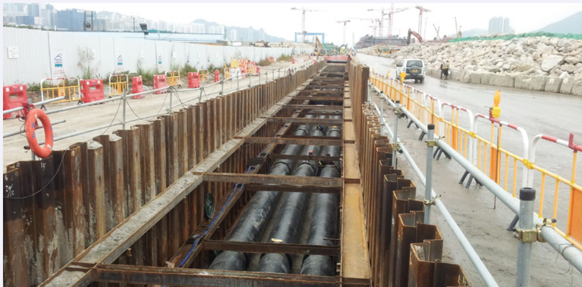
Constructing the Kai Tak District Cooling Systems
