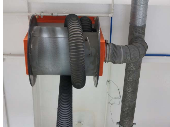
Guide the Exhaust from Vehicle to Outdoors via an Exhaust Hose
