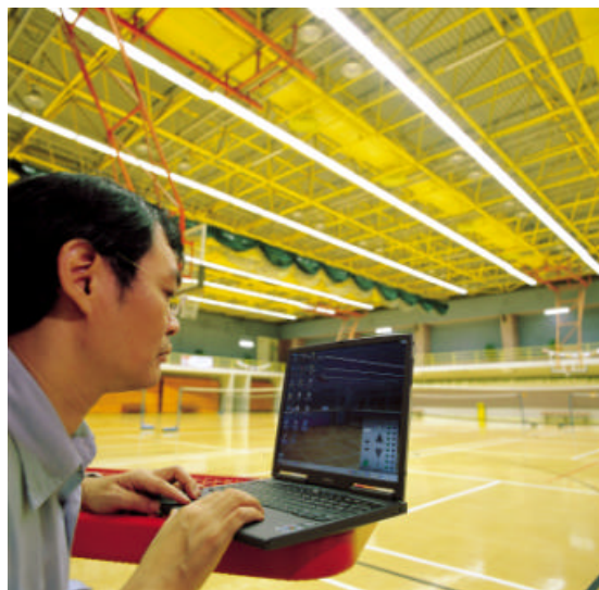
Fig. 5: New lighting control system being programmed
