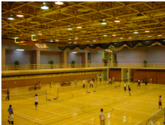
Fig. 1: Existing lighting installations with HID lamps at KBIGH
