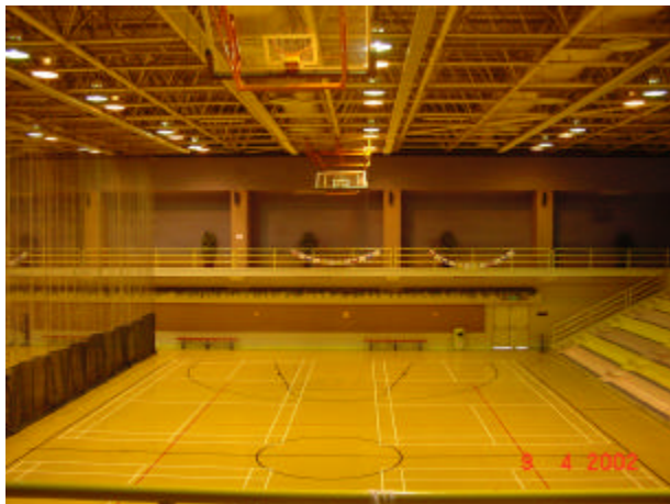
Fig. 9: Existing lighting environment with HID lamps in Kowloon Bay Indoor Games Hall
