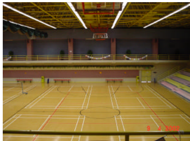
Fig.10: New lighting environment of the High Output T5 Lighting in Kowloon Bay Indoor Games Hall
