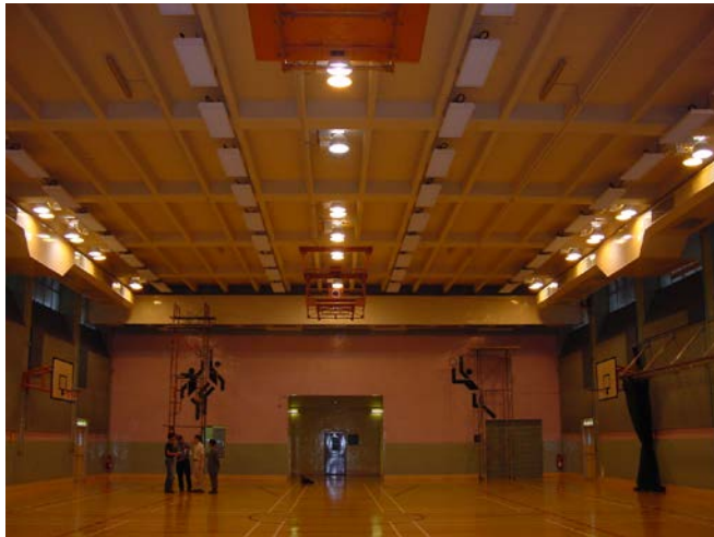
Fig. 2: Existing lighting environment with HID lamps
