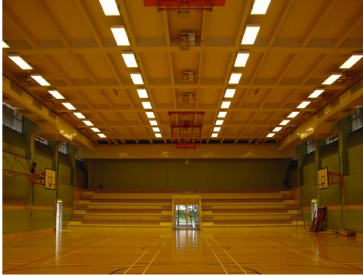
Fig. 6: Visual environment of the new T5 lighting at EKT Indoor Game Hall
