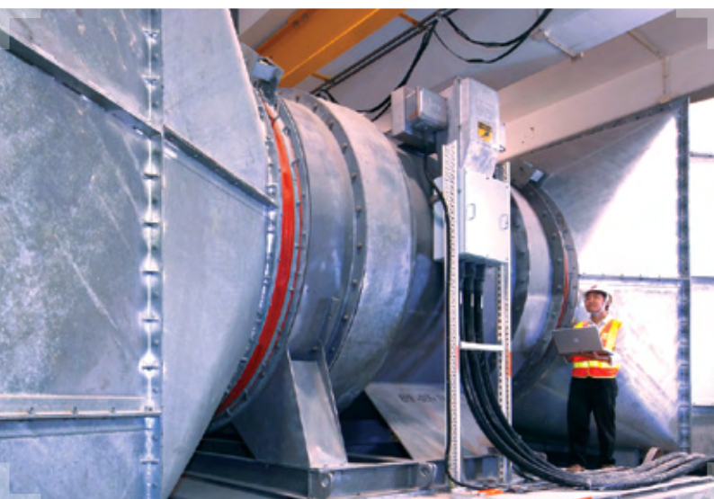
技術人員為八號幹線南灣隧道檢查通風系統。 Technical staff checking the ventilation system at Nam Wan Tunnel of Route 8.
