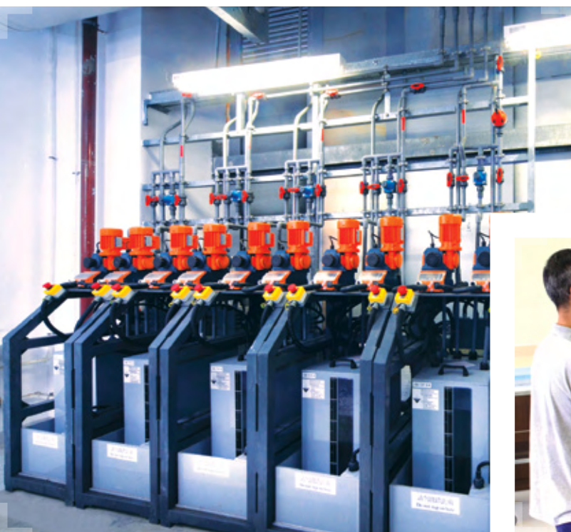
瑪嘉烈醫院醫管局傳染病中心的污水消毒系統。 The Toilet Waste Disinfection System installed at the Hospital Authority Infectious Disease Centre of the Princess Margaret Hospital.
