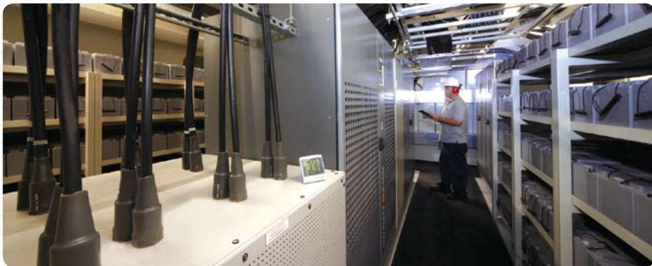
為廉政公署檢查一個雙重不間斷電源系統，確保系統在完成提升工程後可持續提供可靠的電力供應給電腦系統。 Checking a dual uninterruptible power supply system of ICAC to ensure the power supply reliability for computer systems after a major upgrade.
