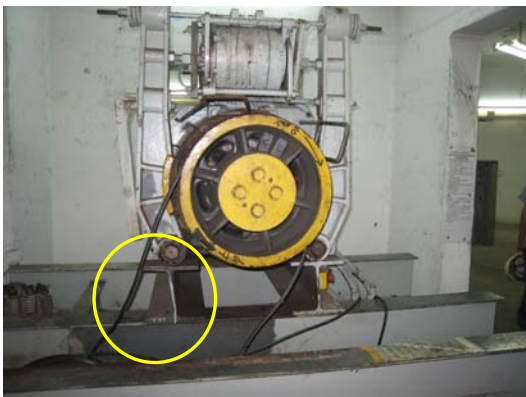
Figure 5A – I-beams of lift motor were deformed.
