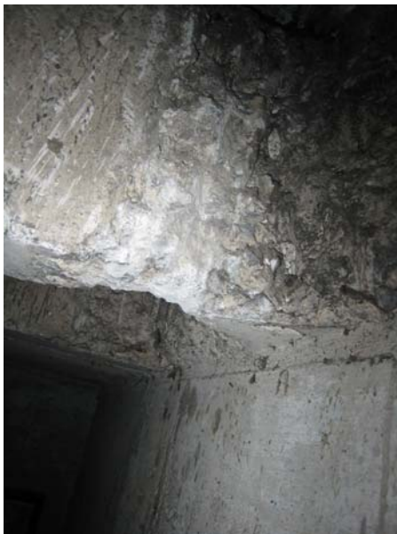
Figure 7 – Concrete slab with new abrasion marks.
