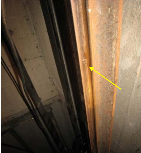
Figure 9 – Intermittent scratch marks on guide rail.
