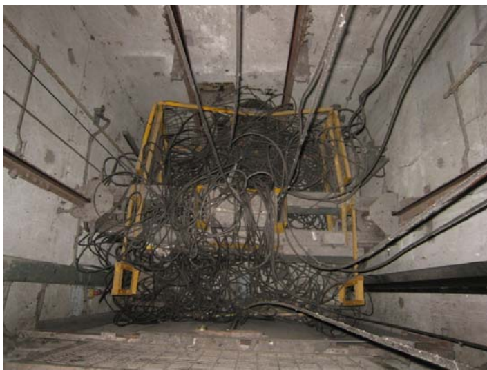
Figure 1 – Lift No.L32 car top and suspension ropes.
