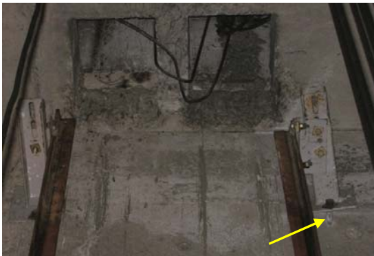
Figure 11 – Deformation of counterweight rail bracket (on the right hand side when looking into the lift shaft from 35/F landing)
