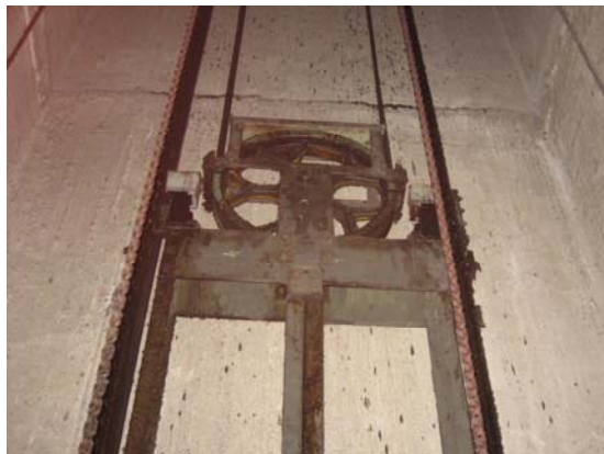
Photo 4 – No damage found from the counterweight.
