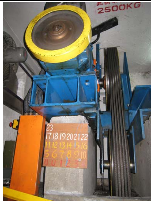
Photo 4 – No damage was found in L2 main drive unit.
