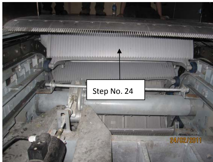
Photo 2 – First jammed step (step no. 24) below the comb plate at upper landing.
