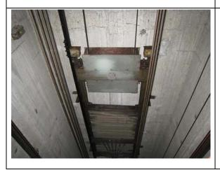
Photo 3 – No damage found from the counterweight.
