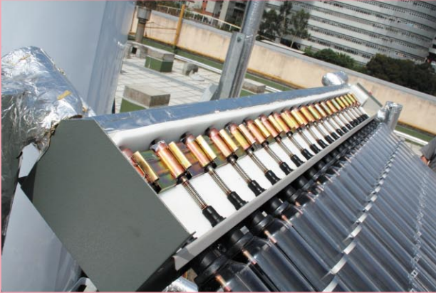
歧管夾着真空熱管 Evacuated Heat-pipes Clipped onto Manifold
