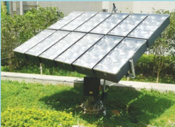
機電工程署大樓外的聚光光伏系統 The concentrated photovoltaic system (CPV) outside EMSD Headquarters building
