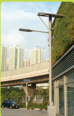
安裝於北廠的太陽能燈 The solar lamp installed in North Plant
