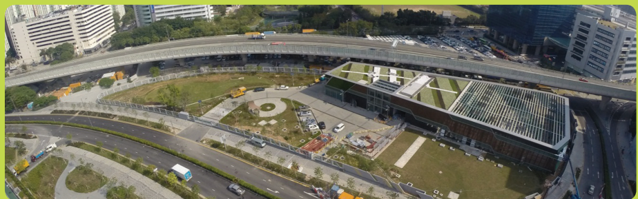
啟德區域供冷系統(北廠)的綠化面積比率逾六成 The greening ratio of Kai Tak District Cooling System (North Plant) is above 60%
