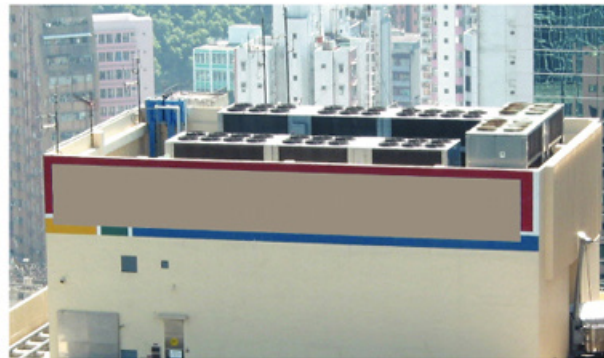
氣冷轉作水冷可節省能源 Conversion of air-cooled A/C to water-cooled A/C can achieve saving
