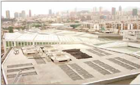
又一城屋頂的冷卻塔 Cooling towers on the roof of Festival Walk
