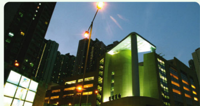
房屋委員會的彩明商場是首幢根據能效守則註冊的建築物 Housing Authority's Choi Ming Shopping Centre is the first building making use of the Performance-based Building Energy Code for registration under the Scheme
