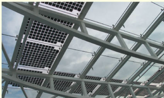
觀景台的光伏玻璃單元 The PV glass units on the viewing gallery
