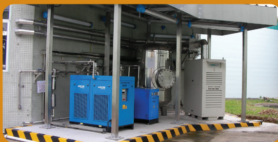
圖2.元朗污水處理廠的微型渦輪發電機系統 Figure 2. Micro-turbine generator system at Yuen Long Sewage Treatment Works
