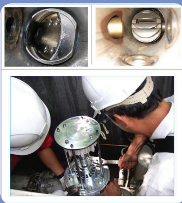
內聯閉式水力發電系統 In-line hydropower harness device
