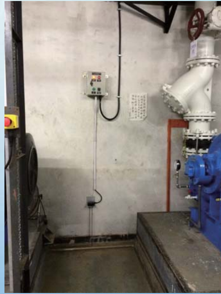
安裝水濕探測系統 WATER LEAKAGE DETECTION SYSTEM
