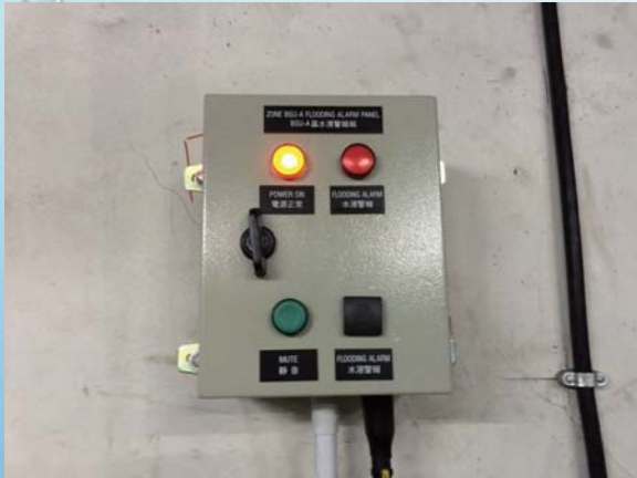
安裝水濕探測系統 WATER LEAKAGE DETECTION SYSTEM
