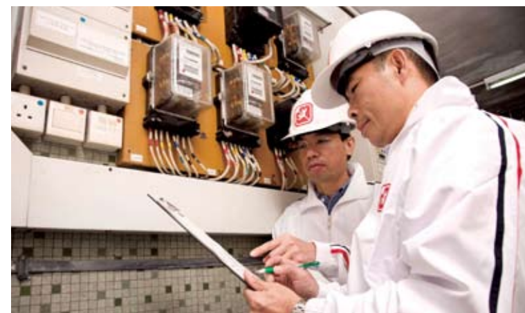
Regular inspection of fixed electrical installation in buildings is a vital task of our inspectorate staff.
