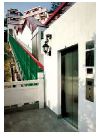
An outdoor "inclined" lift in Sha Tin to suit the terrain.
