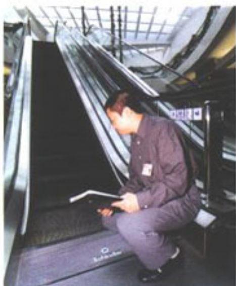
Inspecting an escalator in a shopping arcade
