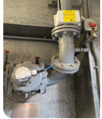
Figure 6: Smart Gas Meter for Commercial Kitchens / Industrial use
