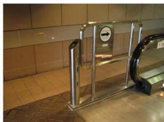
Sufficient clearance space is required for installing sensor pole and barriers 安裝感應器及欄柵需要有足夠的空間
