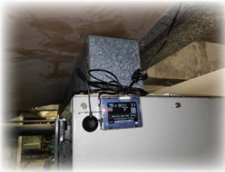
位於馬鞍山游泳池監測過濾系統的感測器 LoRa sensor for filtration pump system monitoring at Ma On Shan Swimming Pool
