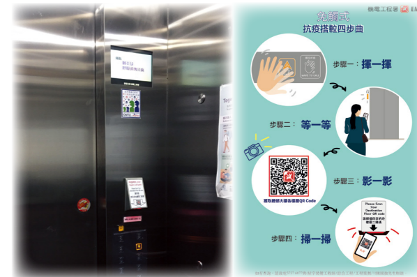
部門已加裝二維條碼掃描器作升降機內非接觸式樓層控制 Addition of QR code scanner as contactless means to assign the designated floor inside the lift car
