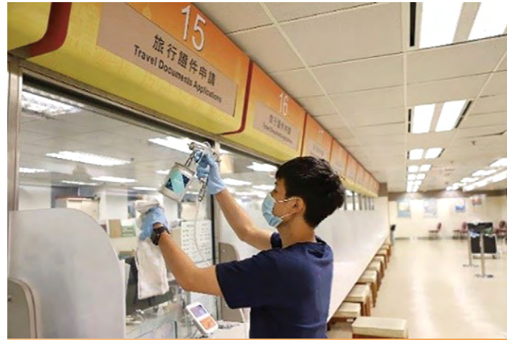
為灣仔入境事務大樓的設施、升降機及升降機大堂噴塗已霧化的納米光觸媒消毒塗層 A disinfection coating of atomised photocatalytic nanoparticles is sprayed on the facilities, lifts and lift lobbies at the Immigration Tower in Wan Chai
