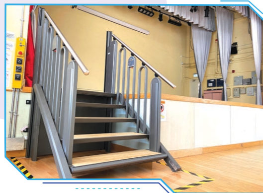
新型升降台日常可作梯級使用，並附有按鈕可操控平台升降輪椅 The new stairlift on standby may be used as a staircase, while it also has buttons at the side for controlling the transfer of wheelchairs up or down
