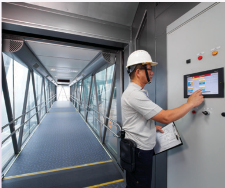
在新啟德郵輪碼頭，我們的工作人員透過船橋內的控制屏測試及校驗登船橋的操作。 At the new Kai Tak Cruise Terminal, our staff conducts testing and commissioning of the Seaport Passenger Boarding Bridge operation through a control console inside the Bridge.
