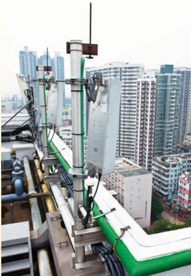
九龍政府合署及其他地方已安裝消防處數碼集群無線電系統的天線，以提升無線電覆蓋範圍及通訊效率。 Antennas for Fire Services Department's Digital Trunked Radio System were installed at various locations, for example the Kowloon Government Offices, to enhance radio coverage and communication efficiency.
