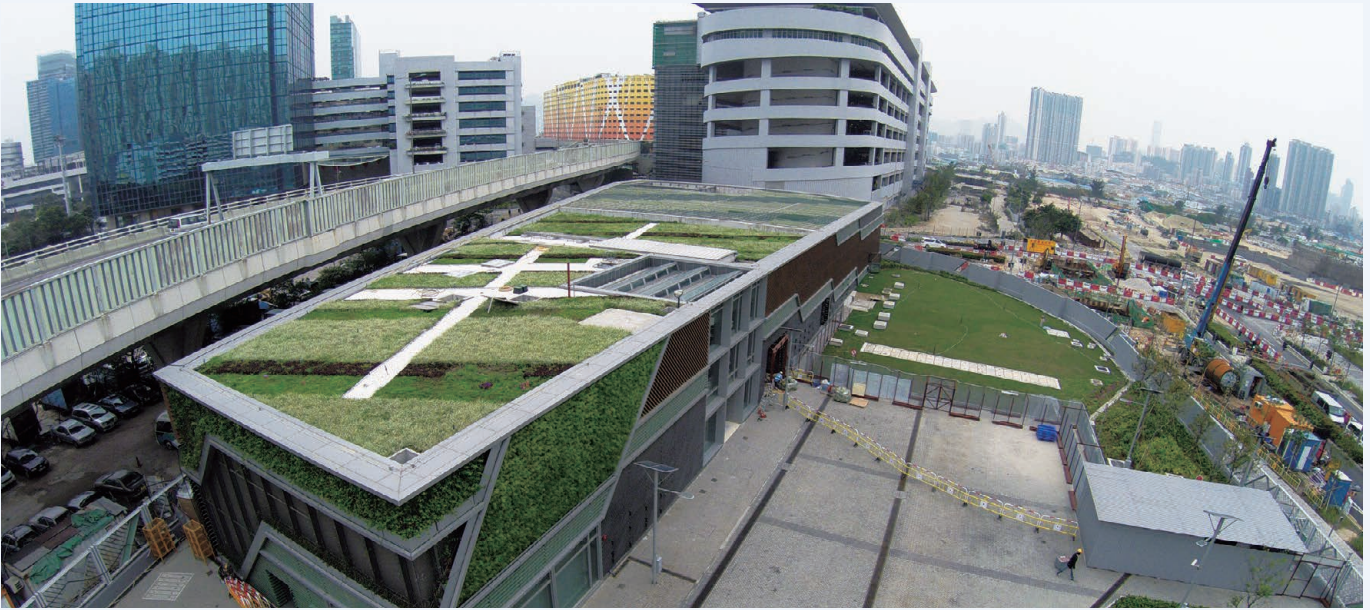
啟德發展區區域供冷系統第一和第二期工程已如期完成，而第三期（A組）工程也進展良好。 Phases I and II of the Kai Tak District Cooling System were completed on time and Phase III (Package A) works are making good progress.
