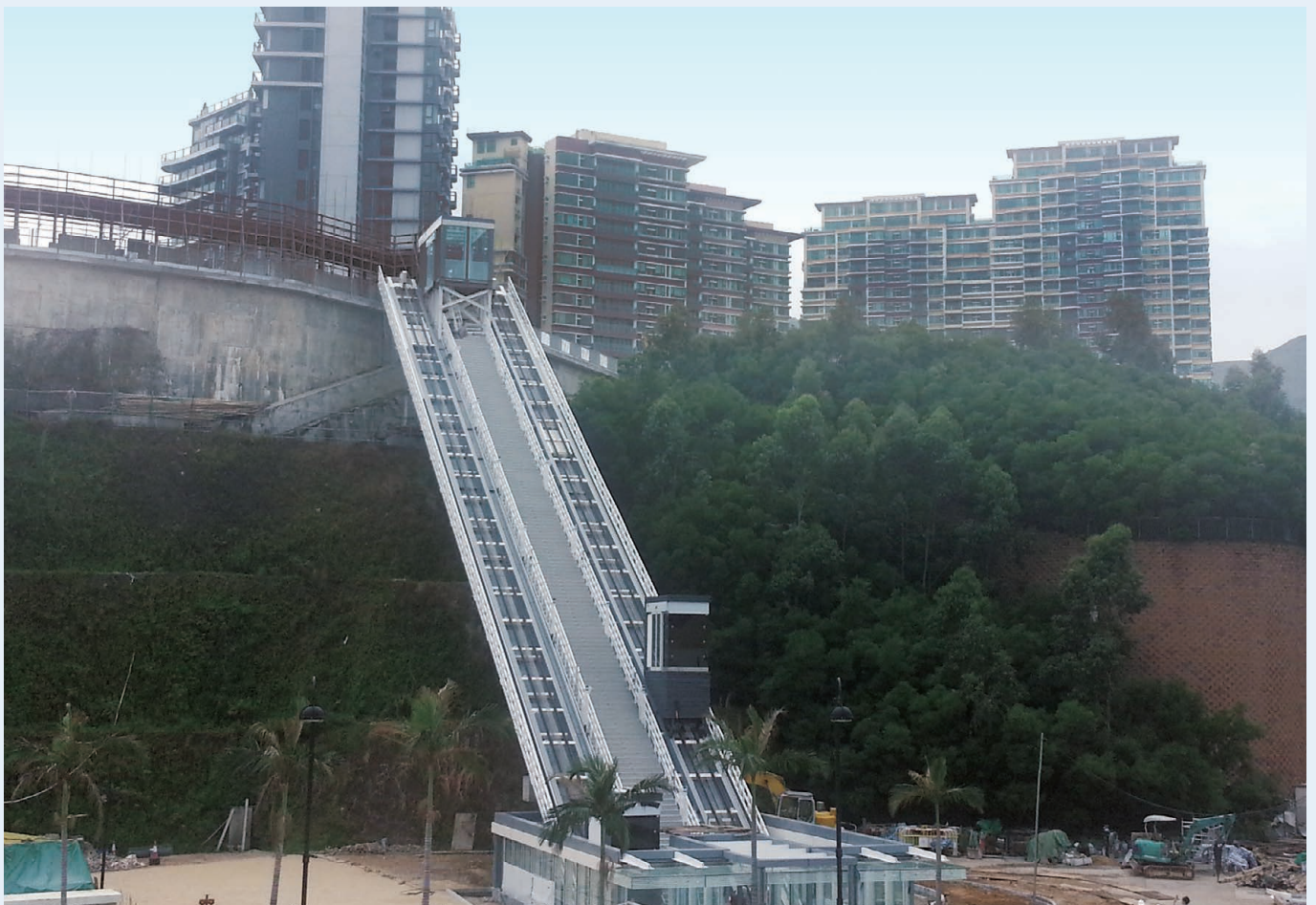
近期引入香港的傾斜式升降機，安裝於愉景灣，是新類型的升降機。 An "inclined" lift in Discovery Bay, a new lift type recently introduced into Hong Kong.
