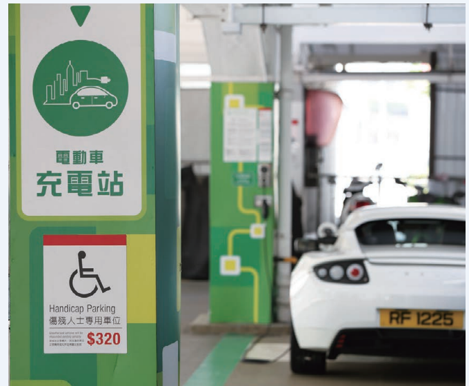
全港各政府停車場已安裝了約100個中速充電器，它們較標準充電器可縮短充電時間約達六成。 About 100 medium-speed charging points are now available in government car parks. They can reduce charging time by up to 60% compared with standard charging points.
