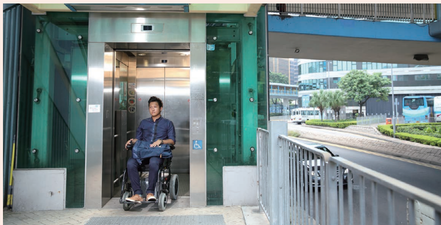
我們提供技術支援予路政署及土木工程拓展署，在行人通道加裝升降機，為市民提供暢通無阻的通道。 We provided technical support to Highways Department and Civil Engineering and Development Department to install lifts at walkways, providing convenient barrier-free access to the public.
