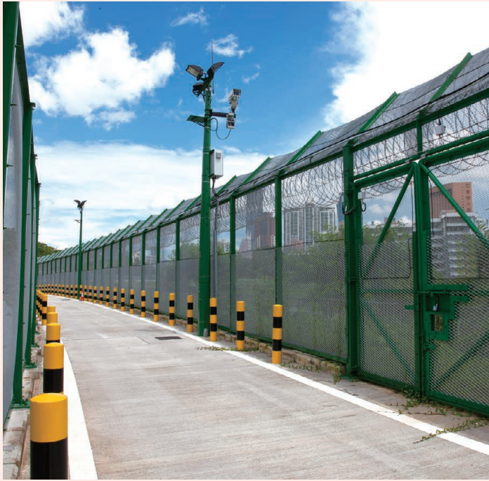
因應實施邊境禁區範圍縮減，我們協助香港警務處在落馬洲路段安裝一套新的邊界圍網保安系統，加強邊境保安。 We assisted Hong Kong Police Force reinforce border security by building a new border fence protection system at Lok Ma Chau section for the implementation of reduction of Frontier Closed Area.
