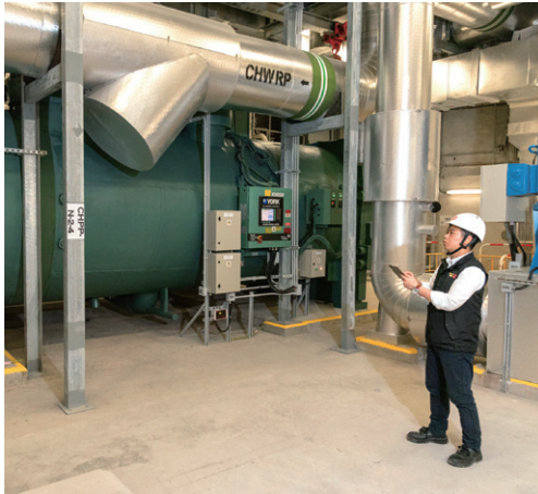
為北廠內的製冷設備進行定期檢查和維修保養。 Regular inspection and maintenance of chiller equipment inside the North Plant.
