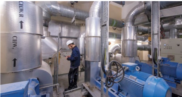
為符合公共衛生檢測中心對室內溫度和濕度的嚴格要求，我們在中心試用自行研發的ChillStream®人工智能製冷機組優化系統，自動調節製冷機組的運作模式，從而節省能源。 To meet the stringent indoor temperature and humidity requirements of the Public Health Laboratory Centre, we trialled our self-developed ChillStream®, an AI-based chiller plant optimisation system, at the centre to automatically adjust the operational mode of its chillers for saving energy.
