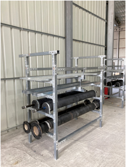
啟德區域供冷系統三號廠房應用了機電裝備合成法，大部分複雜組件都在工廠預製，再於工地裝嵌。這不但加快工程進度，也可避免工程人員在狹窄環境中工作的潛在安全問題。 The Kai Tak DCS Plant No.3 applied the MiMEP method. Most of the complex components were pre-assembled in factories and then assembled at the construction site. This not only accelerated the progress of works, but also avoided potential safety hazards to engineering personnel in cramped working environments.
