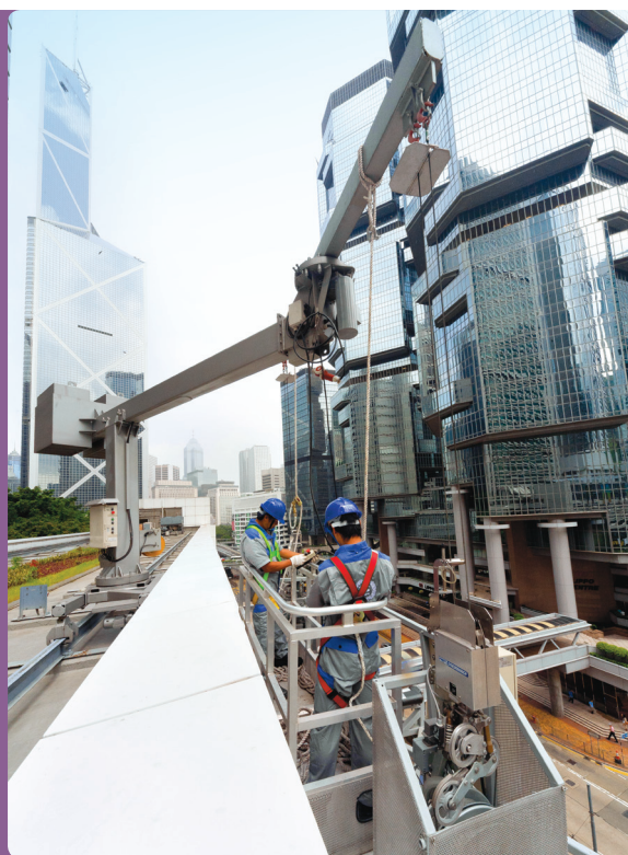
營運基金定期檢查高等法院吊船系統，確保系統安全及可靠運作。 EMSTF conducts regular checks to ensure the safety and reliability of the suspended working platform at the High Court.
