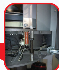
瑪嘉烈醫院使用的氣動輸送系統（左圖）。利用不銹鋼絲桿固定和支撐站台底盤（中圖及右圖）。 The pneumatic tube transport system (left) used at Princess Margaret Hospital and the application of stainless steel rods to fix and support the chassis (middle and right).
