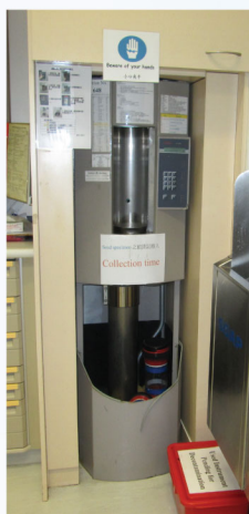
瑪嘉烈醫院使用的氣動輸送系統（左圖）。利用不銹鋼絲桿固定和支撐站台底盤（中圖及右圖）。 The pneumatic tube transport system (left) used at Princess Margaret Hospital and the application of stainless steel rods to fix and support the chassis (middle and right).
