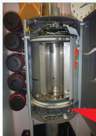
瑪嘉烈醫院使用的氣動輸送系統（左圖）。利用不銹鋼絲桿固定和支撐站台底盤（中圖及右圖）。 The pneumatic tube transport system (left) used at Princess Margaret Hospital and the application of stainless steel rods to fix and support the chassis (middle and right).
