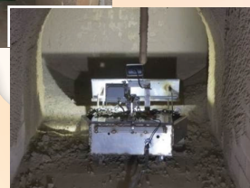
以《遙控剷灰車》在煙道內清理爐灰 Using the remote controlled collector
