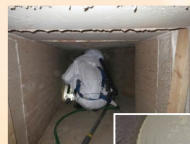
以《遙控剷灰車》在煙道內清理爐灰 Using the remote controlled collector
