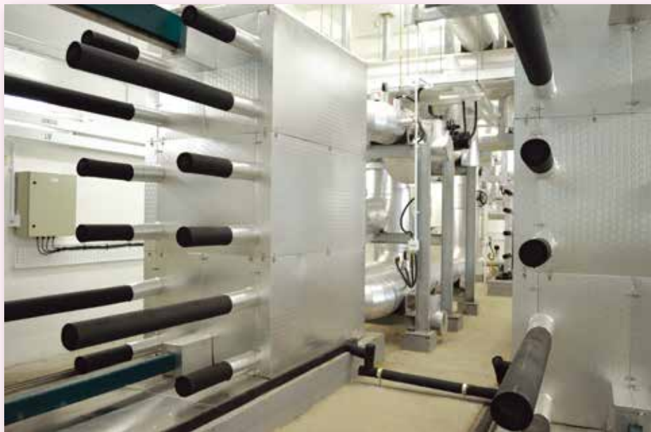
區域供冷系統分站的熱交換器為機電署總部大樓提供冷水，有助大樓每年節省約 15% 用電量。 The heat exchanger of the substation of the DCS provides chilled water for the EMSD Headquarters Building and helps achieve a saving of around 15% in the total electricity consumption.
