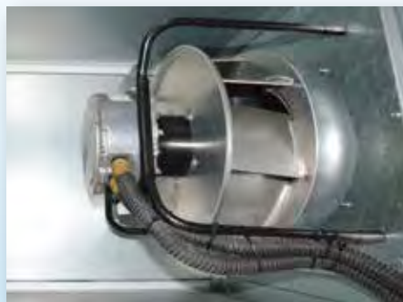
EC風扇的直流電電動機不但耗電量低，而且體積細小。 The DC motor in an EC fan consumes less power and is very compact in size.
