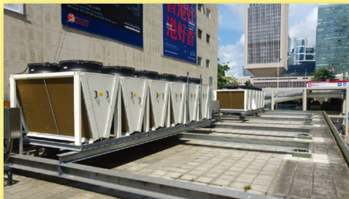
遠距冷凝系統的風冷式冷凝機組安裝於大會堂低座天台，作為應急方案的一部分。 As part of the contingency plan, the air-cooled condensers of the remote condensing system are installed on the rooftop of the City Hall Low Block.
