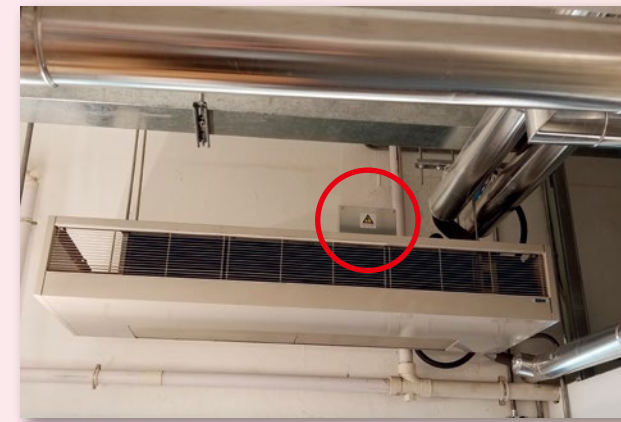
安裝「智能風機盤管控制器」後(見圖示)，當風機馬達以低速運行時，控制器的節能效果尤其明顯。 After installing the Fan Coil Unit Energy Saver (see photo), the energy saving effect is especially noticeable when the fan motor is running at a low speed.
