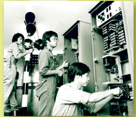
同事維修供電掣櫃 Staff repairing the power supply switchboard
